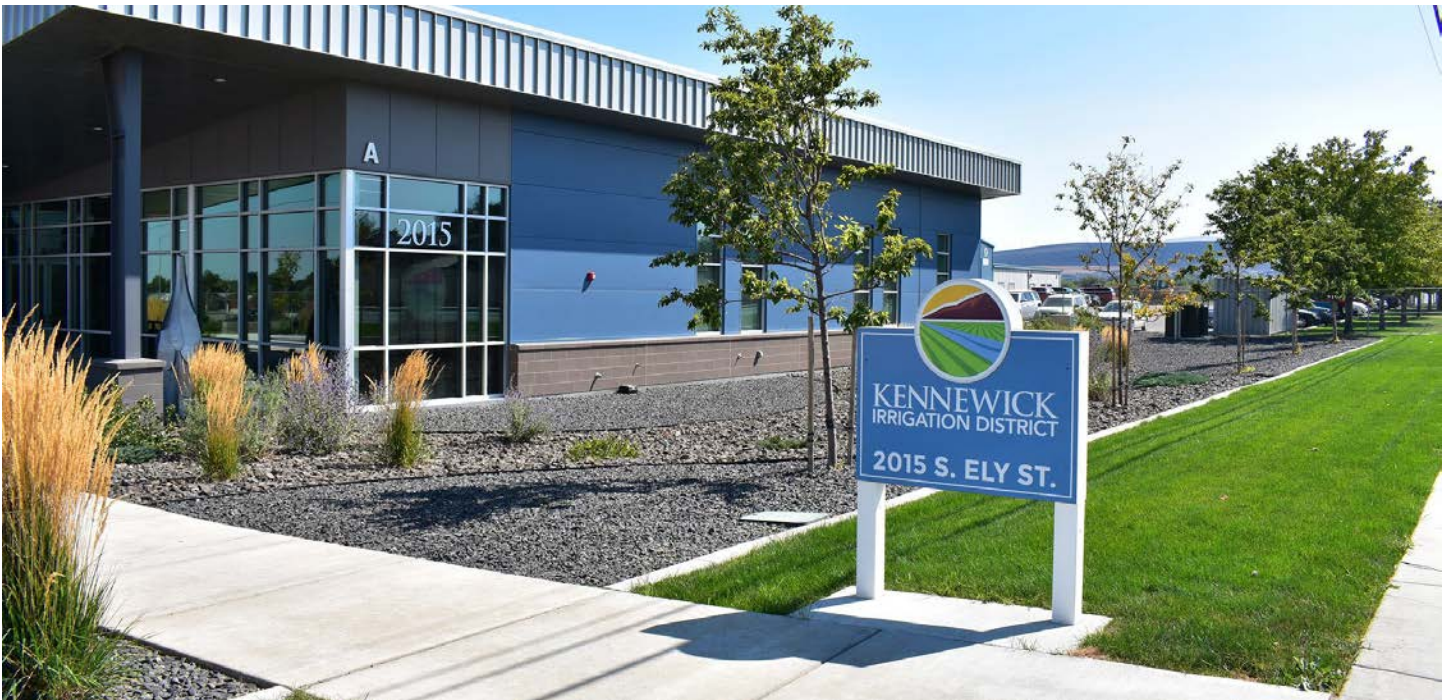
KID headquarters in Kennewick, Washington.
