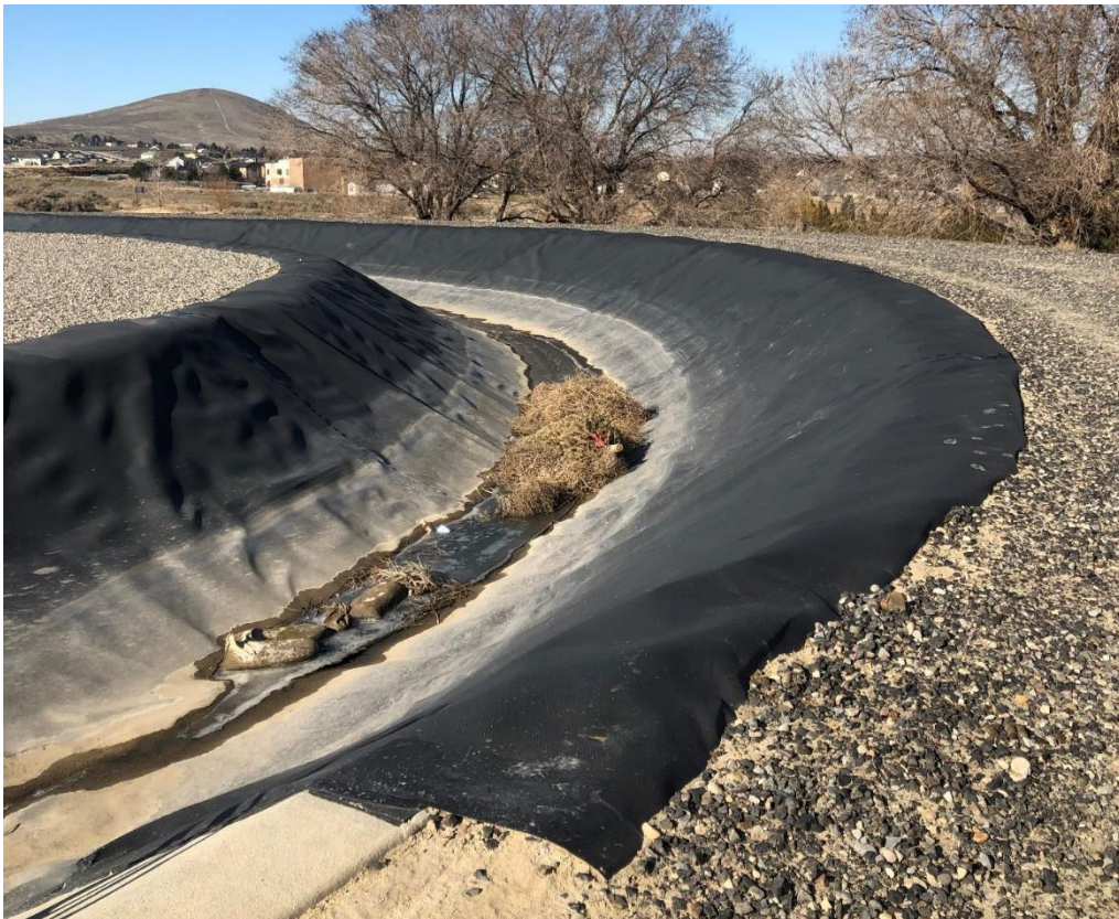
Figure 25. Overview of Badger Lateral East, Near Queensgate Avenue, Aspect: West
