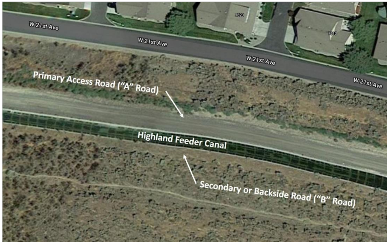
Figure 2. Canal and Adjacent Access Roads (taken from Google Earth)
