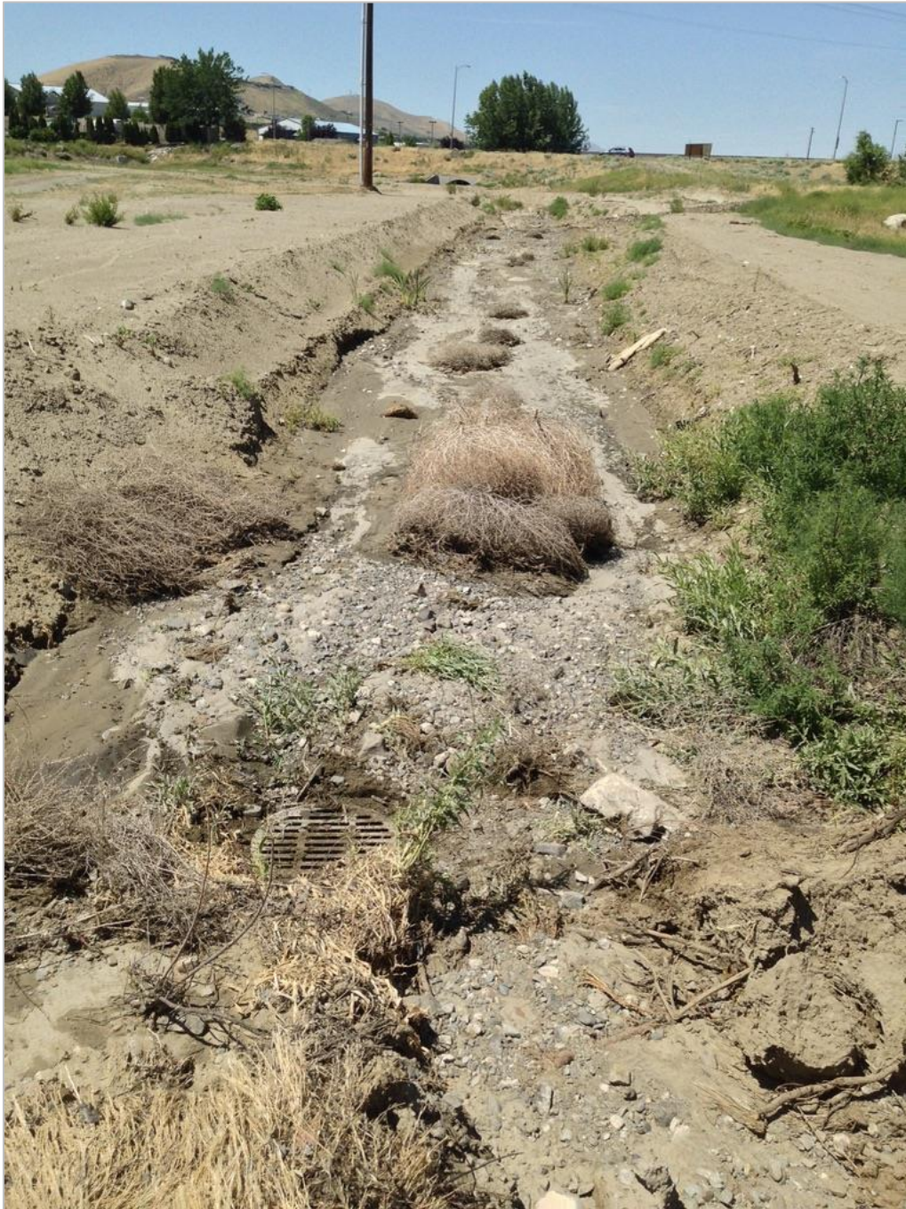
Figure 29. Overview of West Extension Drain, Aspect: West
