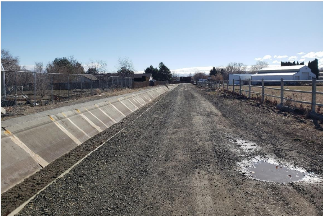
Figure 32. Overview of Highlift Canal, West End, Aspect: East
