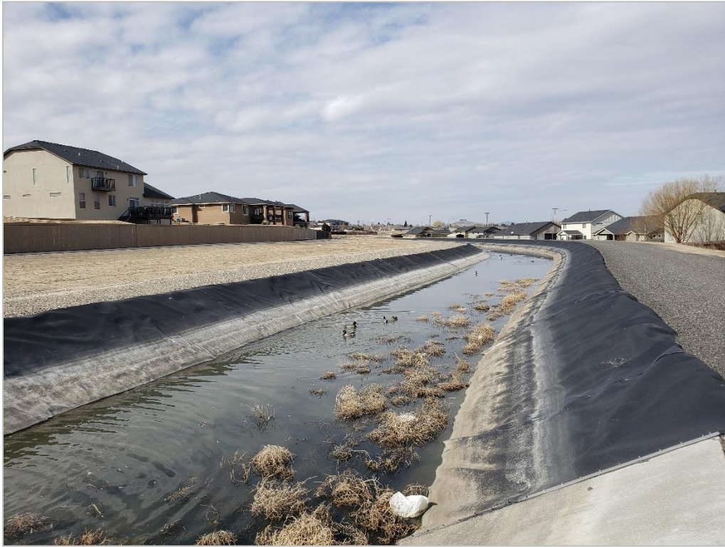
Figure 15. Overview of KID Main Canal Division IV at Turnout 31.5, Aspect: Northwest
