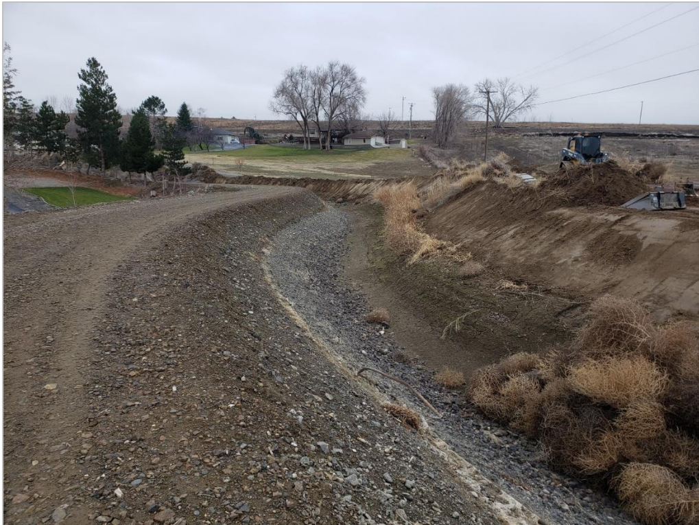
Figure 38. Overview of Highland Feeder Canal, at Turnout 1.1, Aspect: West
