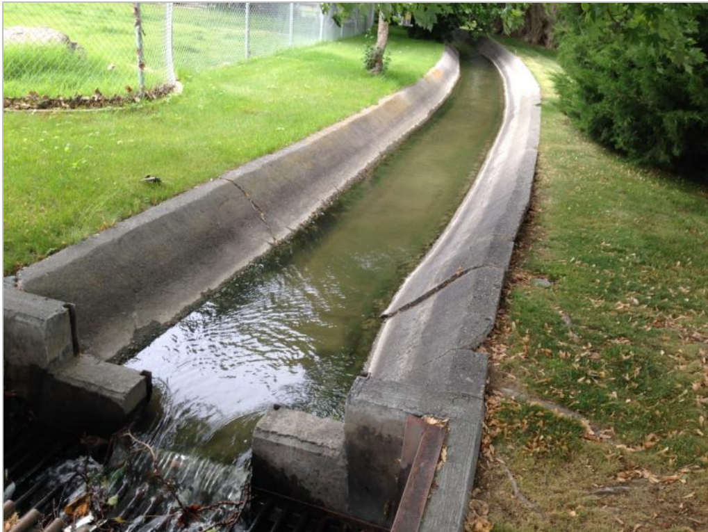
Figure 35. Overview of Lowlift Canal at Its Outlet, Aspect: West
