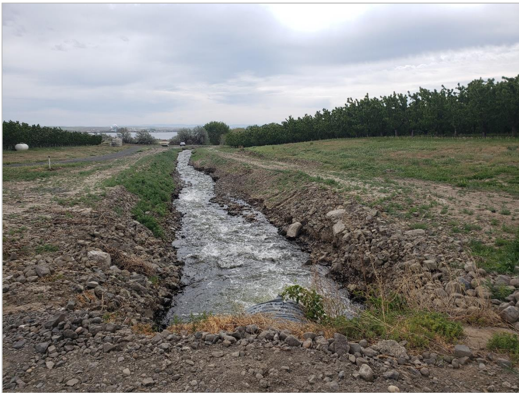
Figure 19. Overview of Hover Wasteway, East End, Aspect: East
