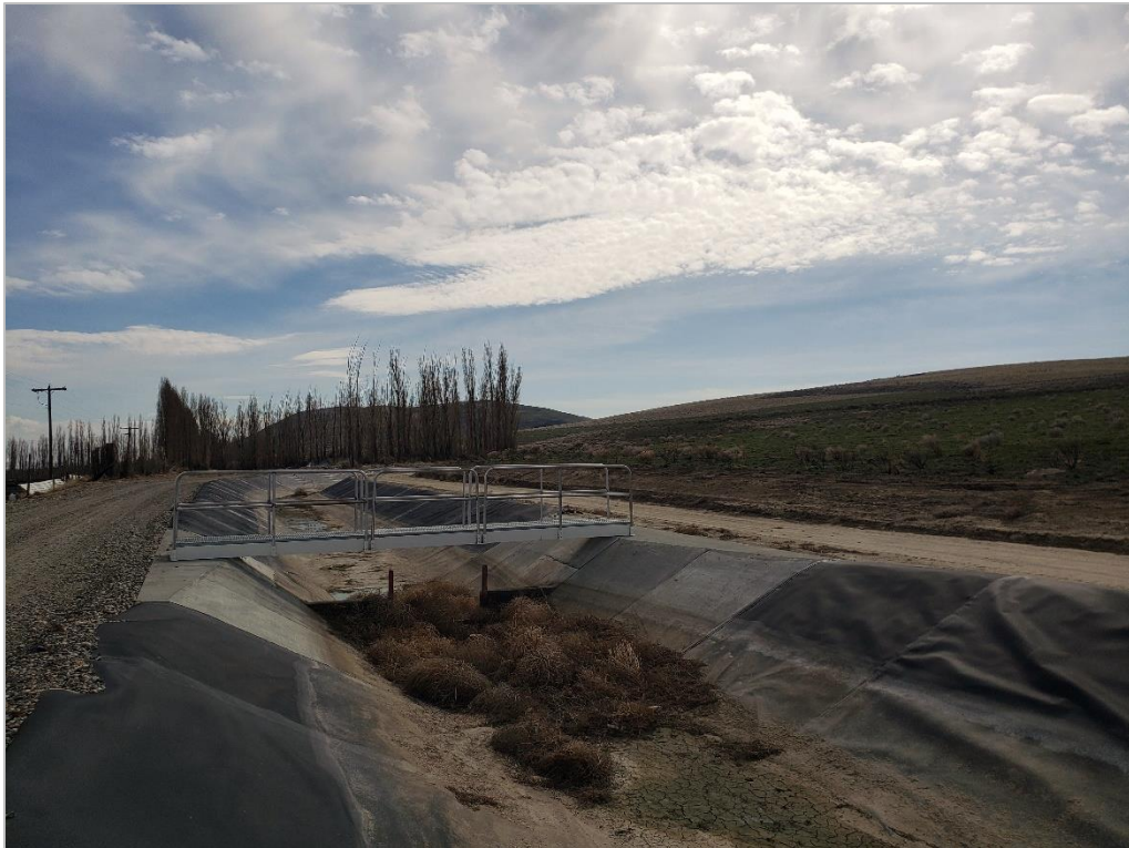
Figure 16. Overview of KID Main Canal Division IV at Turnout 37.6, Aspect: Southeast
