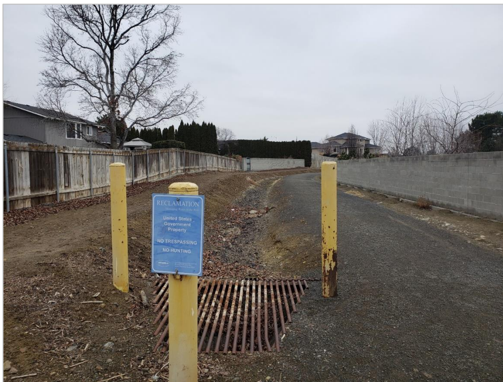
Figure 36. Overview of Highland Feeder Canal, East End, Aspect: West
