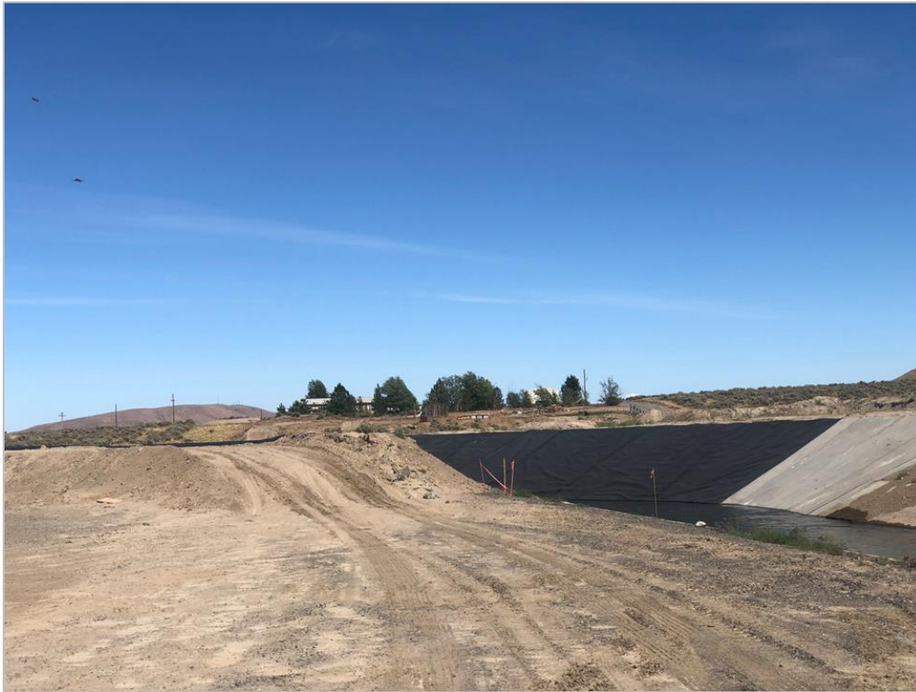
Figure 10. Overview of KID Main Canal Division II, Aspect: East
