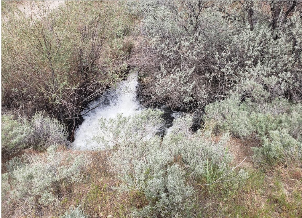
Figure 18. Overview of Hover Wasteway, West End, Aspect: West
