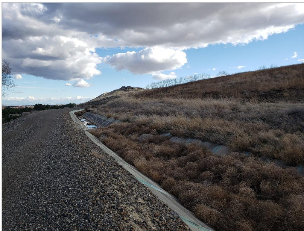
Figure 14. Overview of KID Main Canal Division IV at Turnout 25.8, Aspect: East
