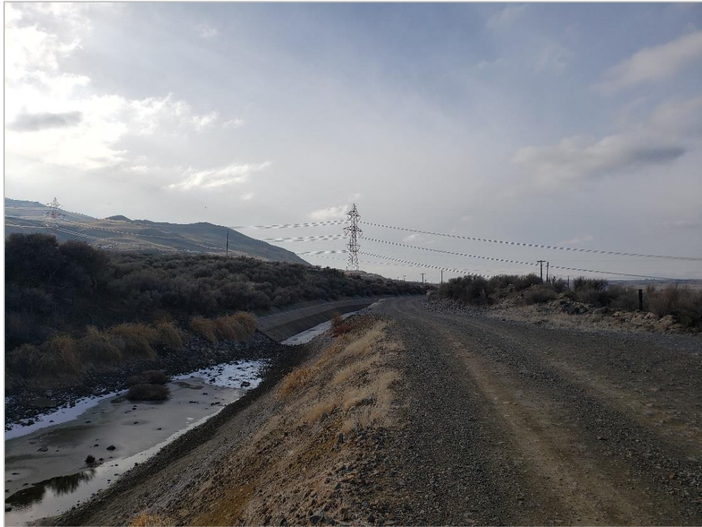
Figure 8. Overview of KID Main Canal Division I at Turnout 2.2, Division I, Aspect: East
