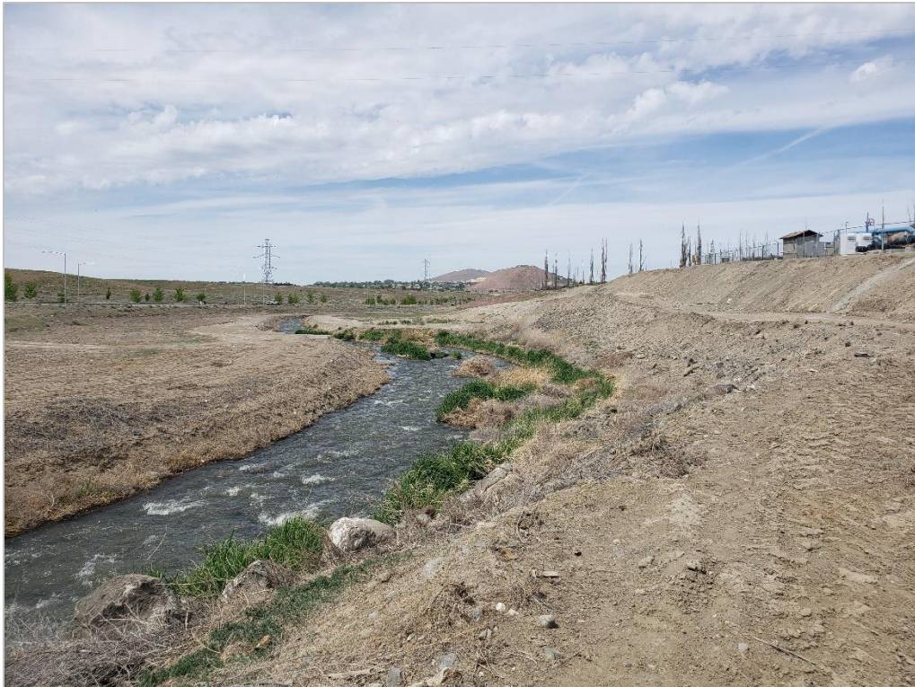
Figure 22. Overview of Amon Wasteway near Amon Pumping Plant, Aspect: West
