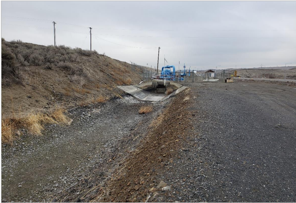
Figure 39. Overview of Amon Pumping Plant and Highland Feeder Canal, Aspect: East
