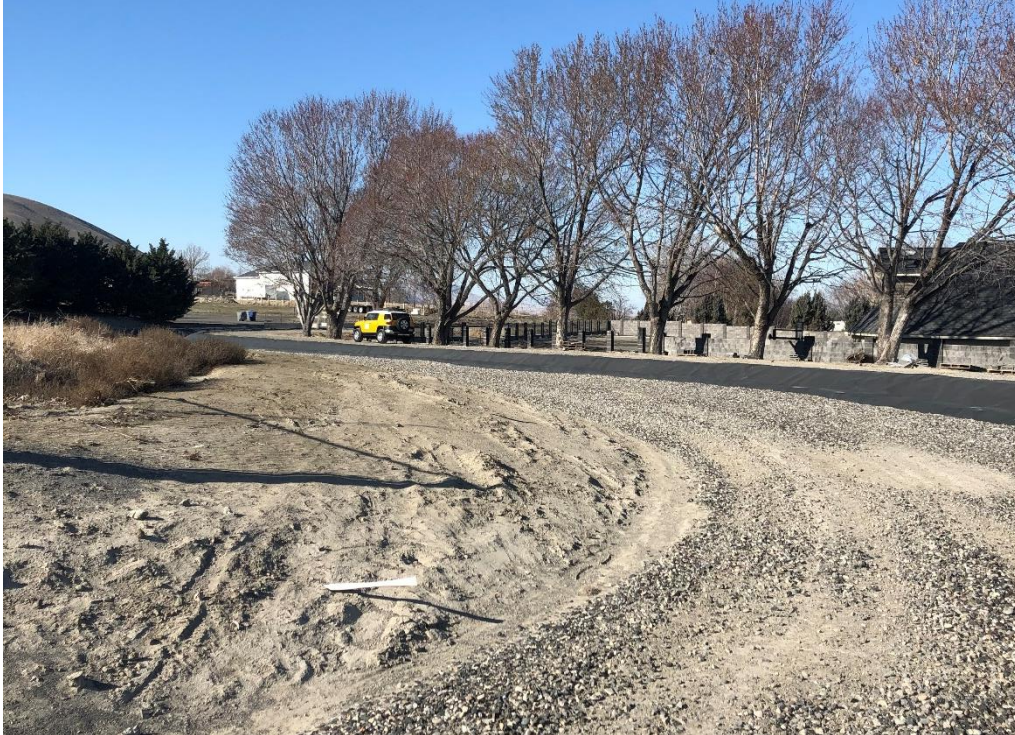
Figure 24. Overview of Badger Lateral East, Near Queensgate Avenue, Aspect: West
