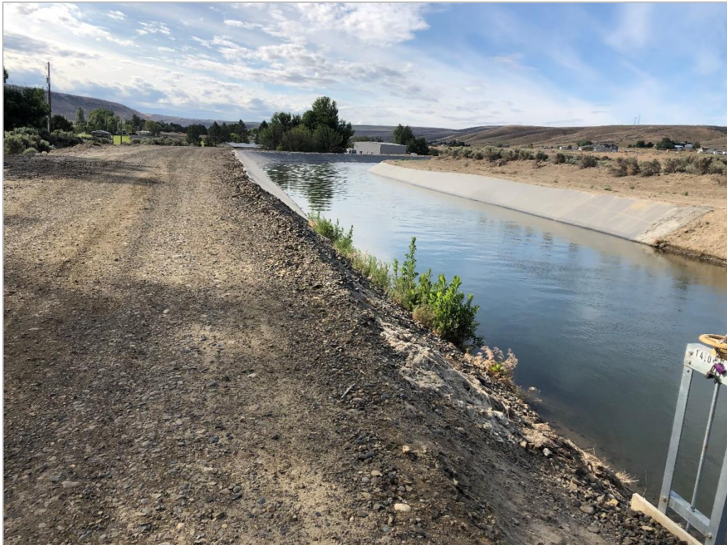
Figure 12. Overview of KID Main Canal Division III at Turnout 14.0, Aspect: East
