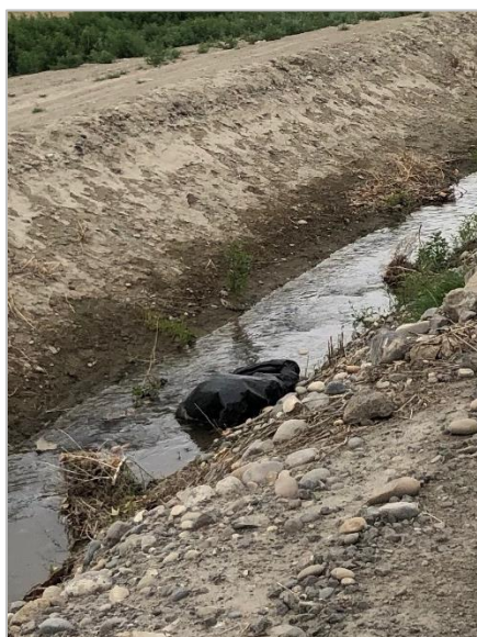
Figure 4. Plastic Trash Bag Debris in Badger West Lateral
