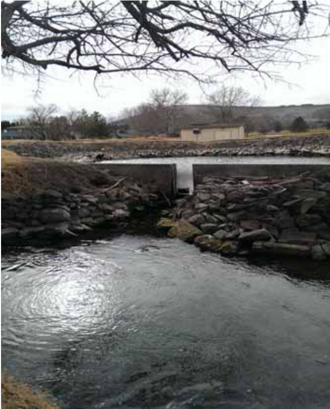
Concrete Flume at WF Amon A, this structure provides a fish passage barrier.
